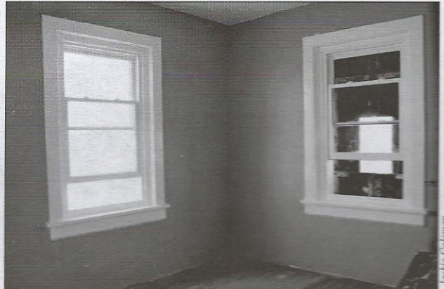
Sheila has already begun restoration of the bedrooms
