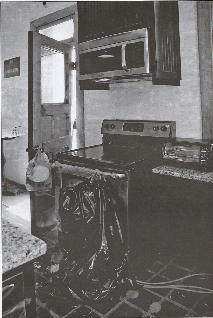
Despite the current lack of running water, waste disposal and electricity, Sheila had just installed all the conveniences of a modern kitchen in the lighthouse.
