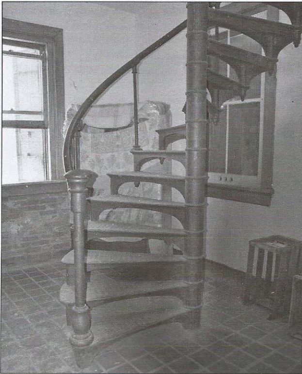
Cast iron stairway leading to the second floor bedrooms
